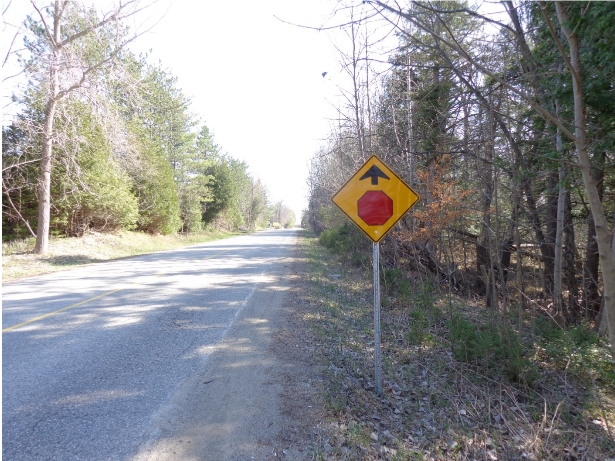
East and Westbound Stop Ahead signs installed 150 metres before Watson Road and Maltby Road intersection.
