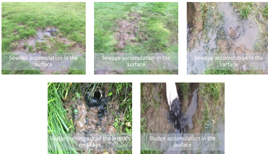
Figure 6-1: Sludge Deposition within the Subsurface Disposal System (Tile Beds)
